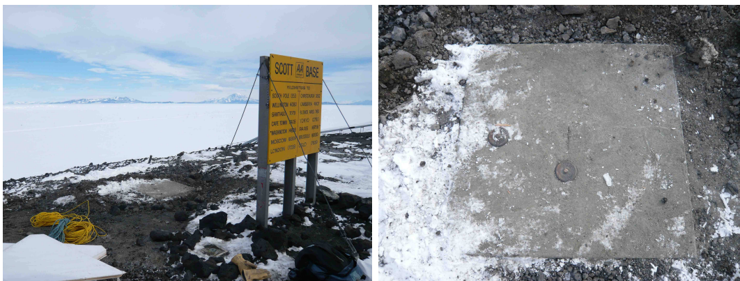
Figure 3.1: Left. Behind the yellow panel, concrete pier holding gravity benchmarks SBG-1 and SBG-3. Right. Gravity benchmarks SBG-1 (centre) and SBG-3 (left).
