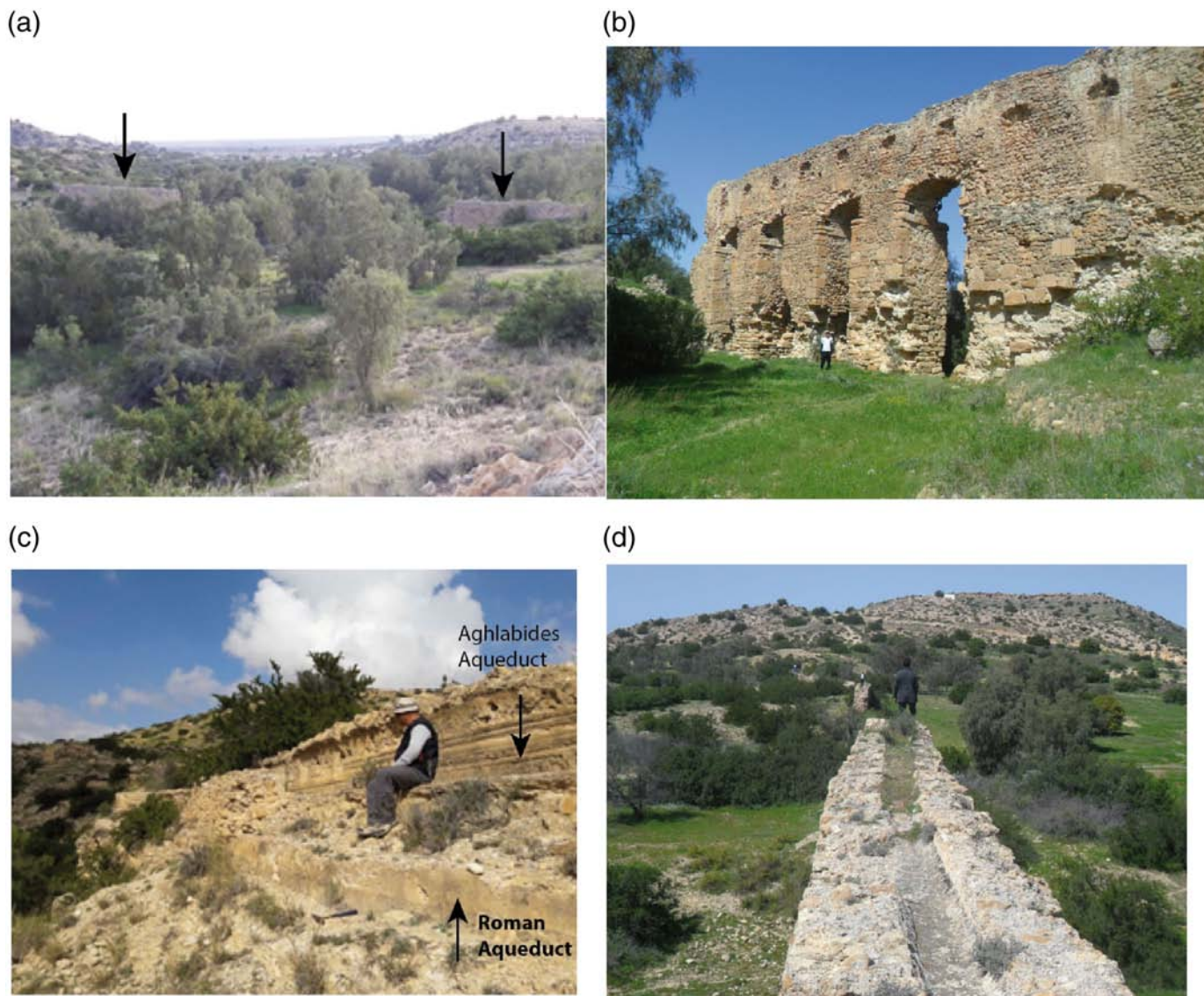
Figure 8. (a) The aqueduct bridge with its edges (arrows) crossing the Cherichira River; (b) ~25-meter-high aqueduct bridge with 2.9 × 2.9 m pillars built during the Roman time in Tunisia (146 B.C.–A.D. 423) and the Aghlabides period (A.D. 800–909); (c) the Roman and Aghlabides Aqueduct exposures; and (d) top of the aqueduct with a canal on the bridge. The color version of this figure is available only in the electronic edition.
